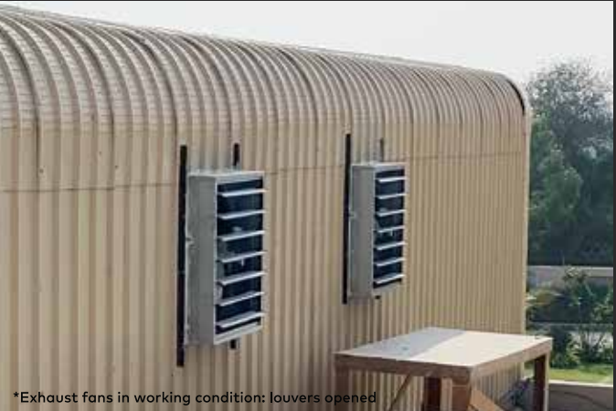
*Exhaust fans in working condition: louvers opened
